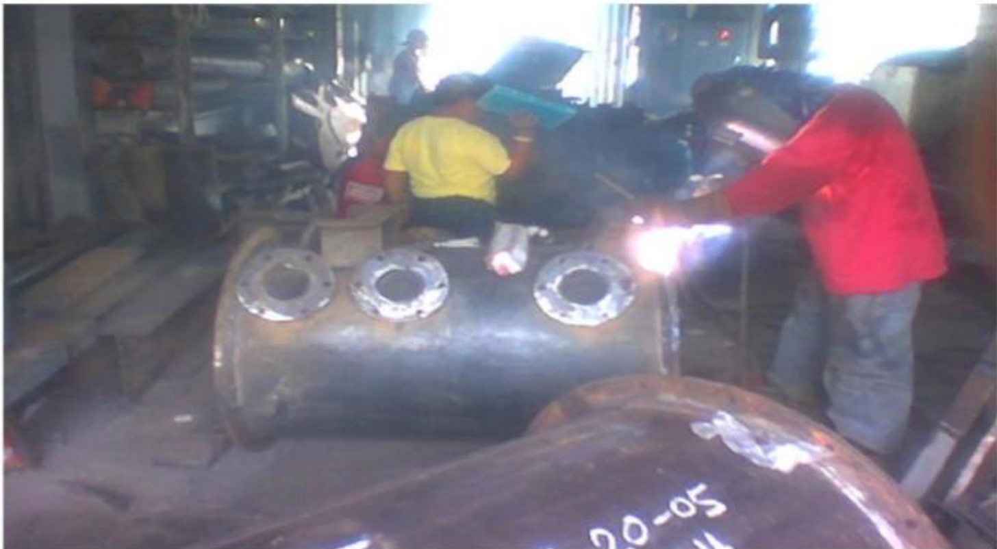
FABRICATION OF GASOLINE CYLINDRICAL TANKS
